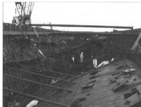
FIGURE-7: WORK ABOARD THE REINFORCED CATALA INSIDE THE SHEET PILE CELL
